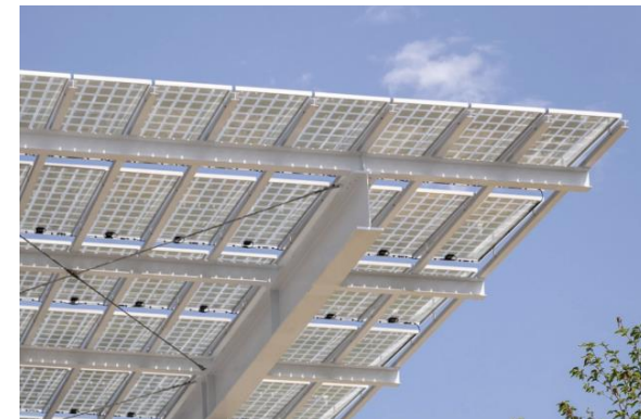
Rudolf and Peter Steiger Architects / CERN
