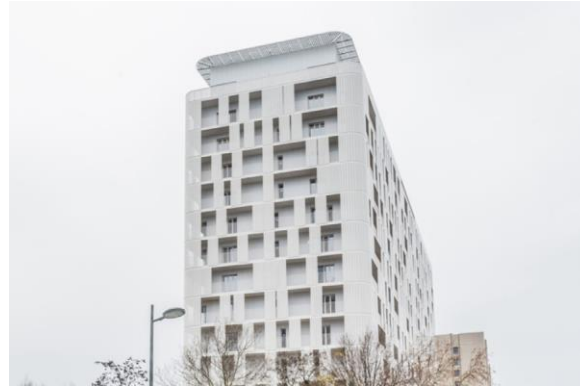
Architectesassoc+ / Leopold Views
