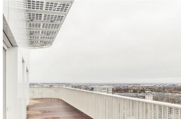
Architectesassoc+ / Leopold Views
