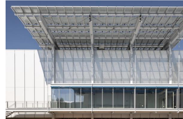
Rudolf and Peter Steiger Architects / CERN
